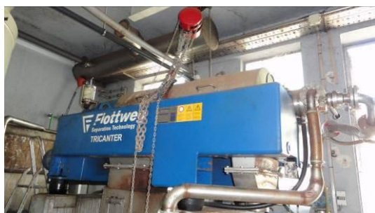
Figure 23 Centrifuge / decanter (WWTP) and Anaerobic filter (biogas)
