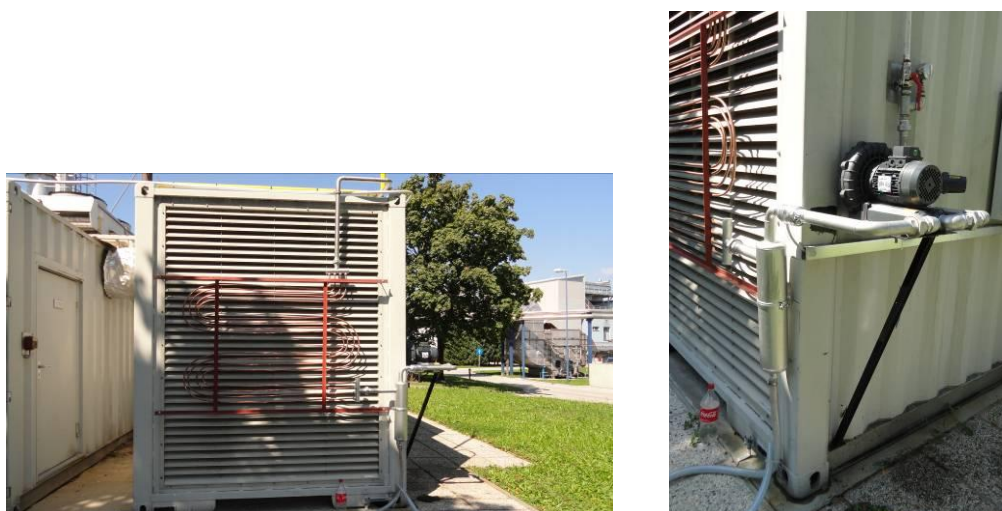
Figure 9 Flue gas heat exchanger and blower with the drain
