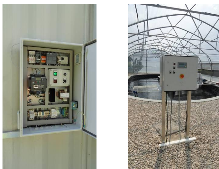
Figure 15 Remote cabinet at the gas-engine and panel at the pond
