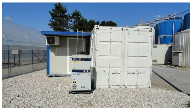
Figure 13 Chiller mounted in front of the equipment containers
