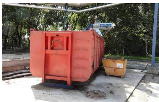
Figure 22 Press Screw Separator and roll-off digestate equalization container
