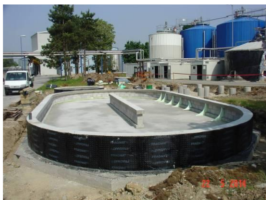
Figure 4 Hydro-insulation and models for the curves
