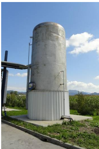
Figure 24 Centrate storage tank (CT1) (ex digestate cooling tank)
