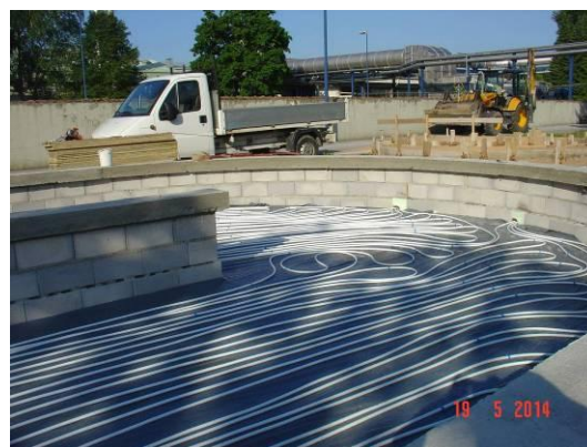
Figure 3 Concrete slab, walls from concrete blocks and under-floor heating pipes
