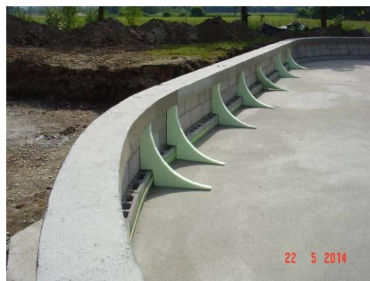
Figure 4 Hydro-insulation and models for the curves
