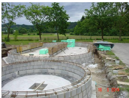
Figure 3 Concrete slab, walls from concrete blocks and under-floor heating pipes
