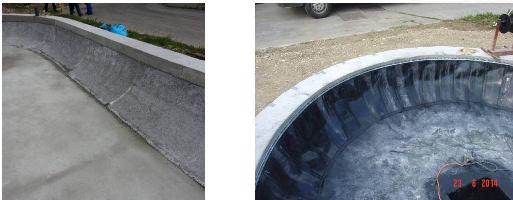
Figure 5 Curves made of EPScrete and PEHD membrane
