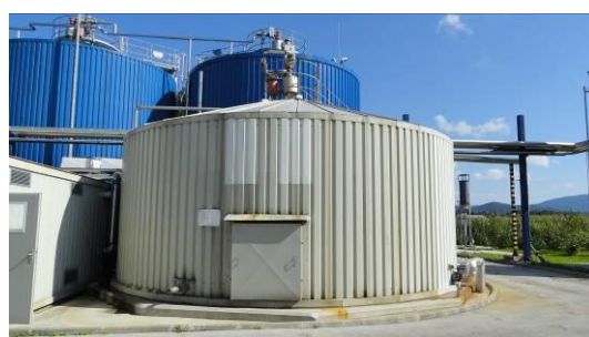
Figure 23 Centrifuge / decanter (WWTP) and Anaerobic filter (biogas)
