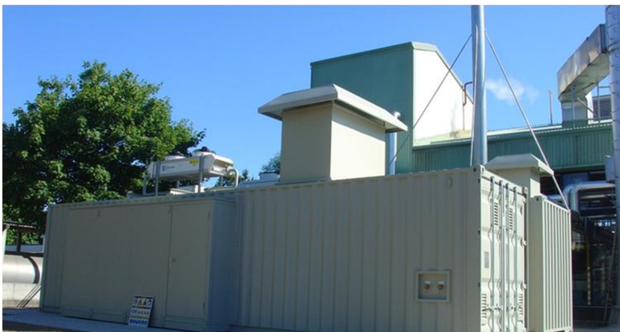
Figure 2 Cogeneration unit, 526 kW at KOTO
