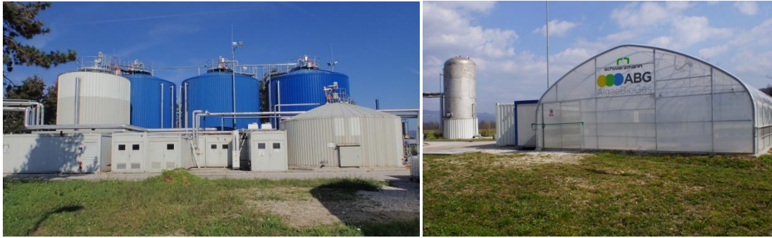
Biogas plant and greenhouse
